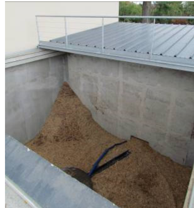
Chaufferie Bois - St Varent
